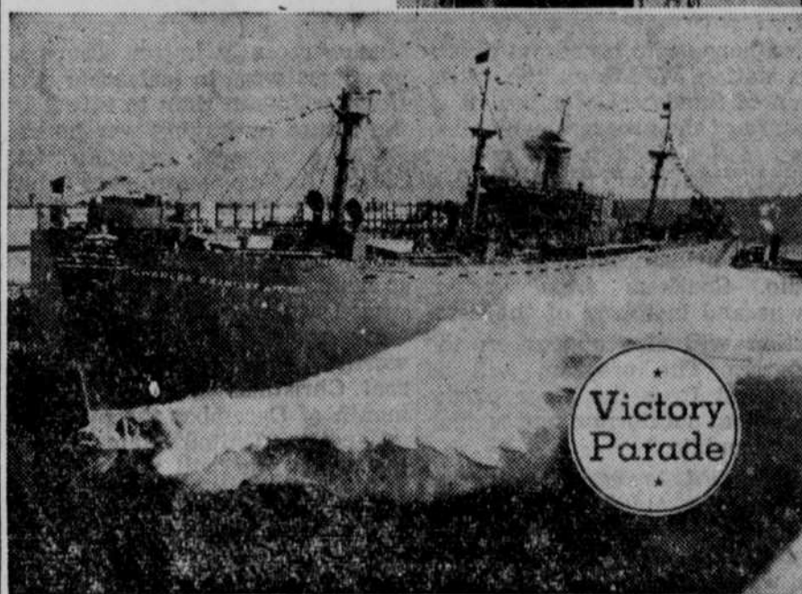
Sidewise launching of an EC-2 Liberty ship at a Gulf Coast port.
