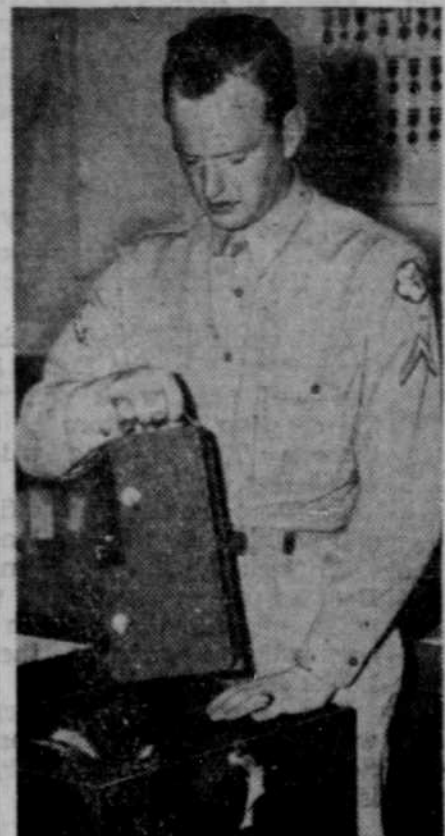
The army and navy soon will inaugurate a new method of microscopically copying letters to soldiers in foreign lands. By means of this method 1,500 letters can be recorded on one reel of film. Three reels are the equivalent of two mail pouches. In this picture Private Erwin Twad-dell removes the camera from the recording machine, for processing before reel is shipped.
