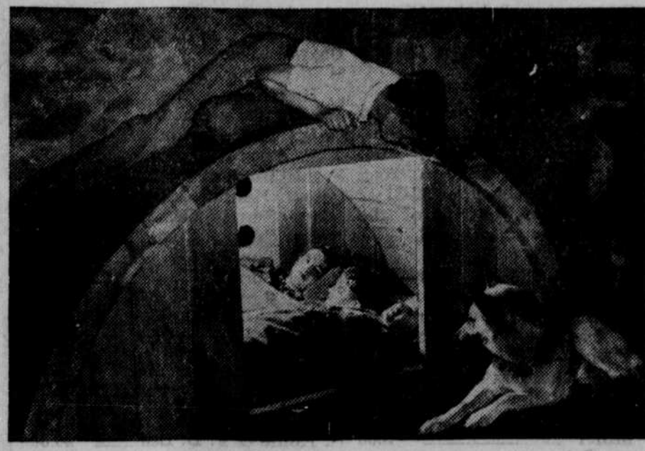
If the brick of this house comes tumbling down, the mother and two children inside this timber air raid shelter would be fairly safe. The heavy timber is easily put together with pegs, contains a double bed and incendiary bomb fighting equipment. The family is bundled in for the night, with one son on top, looking on—and the dog looking in.
