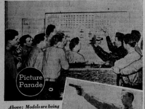
used in range estimation and gunnery training. As the models are built on a scale of an inch to represent six feet, the student can see by looking at a model through a gunsight at a distance of 10 feet how the actual plane would appear at a distance of 240 yards.
