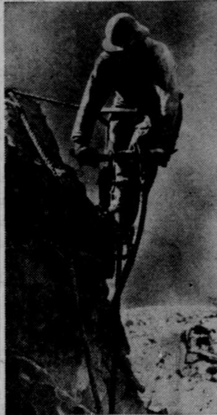
Men who work to increase our supply of electric energy are soldiers, too. Photo shows a jackhammer operator drilling a hole for a dynamite blast on an abutment of Shasta dam, near San Francisco, Calif.
