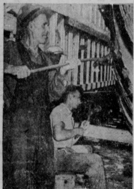
Two workers "dubbing" on the outside of the hull for the exterior planking. They work to a chalkline snapped on the ribs.
