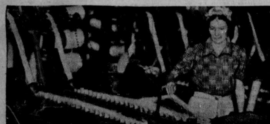
Now in yarn form, rolled on bobbins, the sisal is being spun into a small ball of rope by the girl at the machine.
