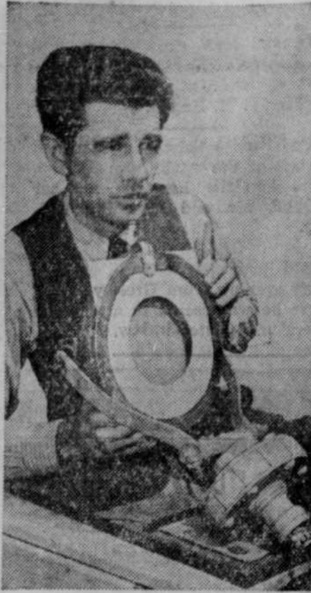
Above: Sun telescope made from an old auto axle. Murray is focusing the solar image on a paper receiver here. Right: At the eyepiece of this homemade telescope he checks up on a few stars. The instrument is made of old water pipes, wood and pieces of mirror. Note how the wood is bound with wire.
