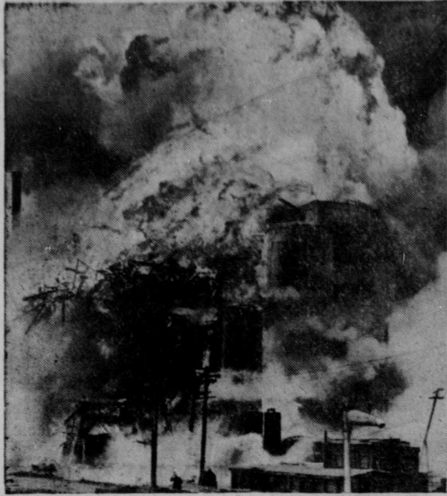
This spectacular picture was taken just as a billow of white hot flame blew off the top of a United States Grain elevator, in Chicago, during a $300,000 fire, of mysterious origin. More than 350,000 bushels of corn were destroyed. Furnace-like heat melted steel girders like butter and drove back firemen.
