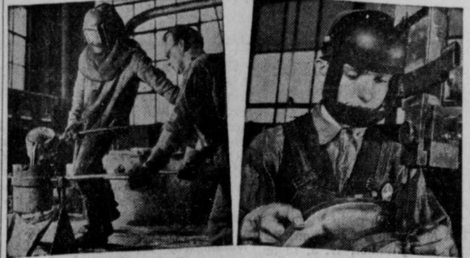
Wearing heavy metal shoes, a fireproof suit and a helmet that looks like a diver's, a worker pours molten metal. This worker is using a band-saw to trim a compound contour formed on a Martin drop hammer. This will go on a bomber.
