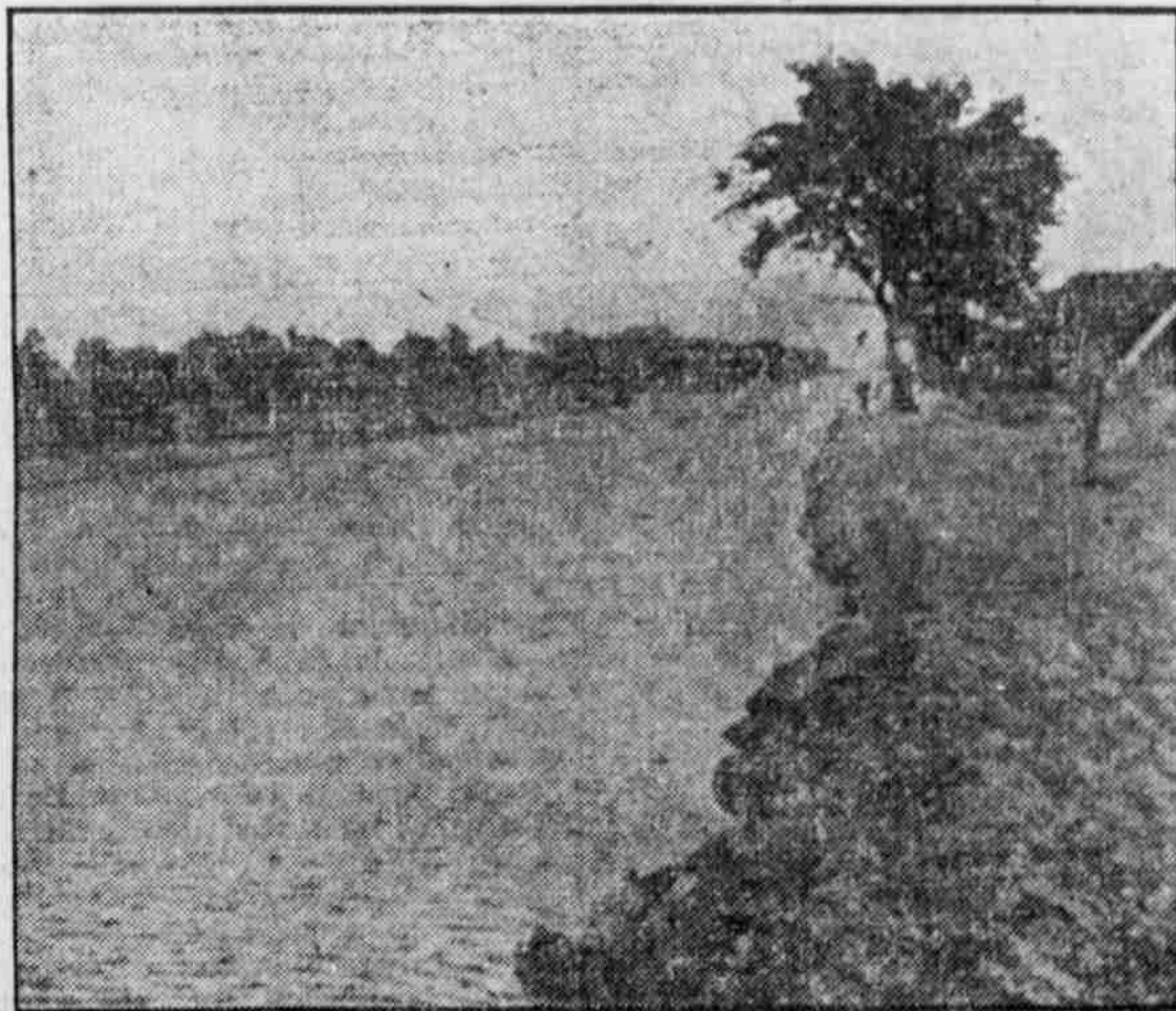
Main Canal of La Lomita Irrigation System
