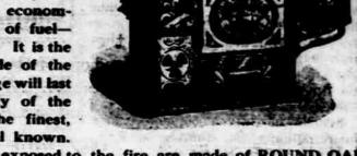
The top and the parts exposed to the fire are made of ROUND OAK cast iron—noted for its strength and durability. The fire front and back are in sections and are extra heavy. The fire box is oval and just exactly the right size. The well fitting hot plates and covers are braced and strengthened differently and better than others. The duplex grates burn successfully
