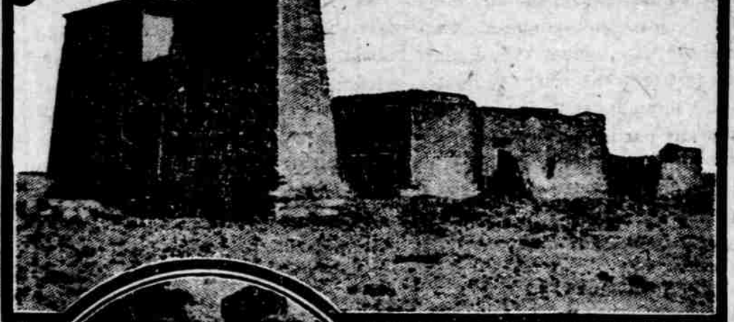
THE TEMPLE AT DANKEH WHICH WILL COLLAPSE UNLESS UNDERPINNED
