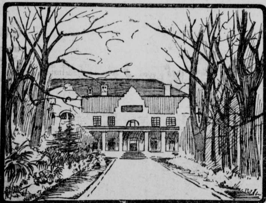
Front of Grootes Schuur, Rondebosch, Near Cape Town.
