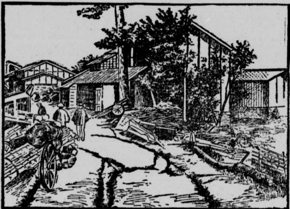
VILLAGE ROAD IN JAPAN, AFTER AN EARTHQUAKE.
