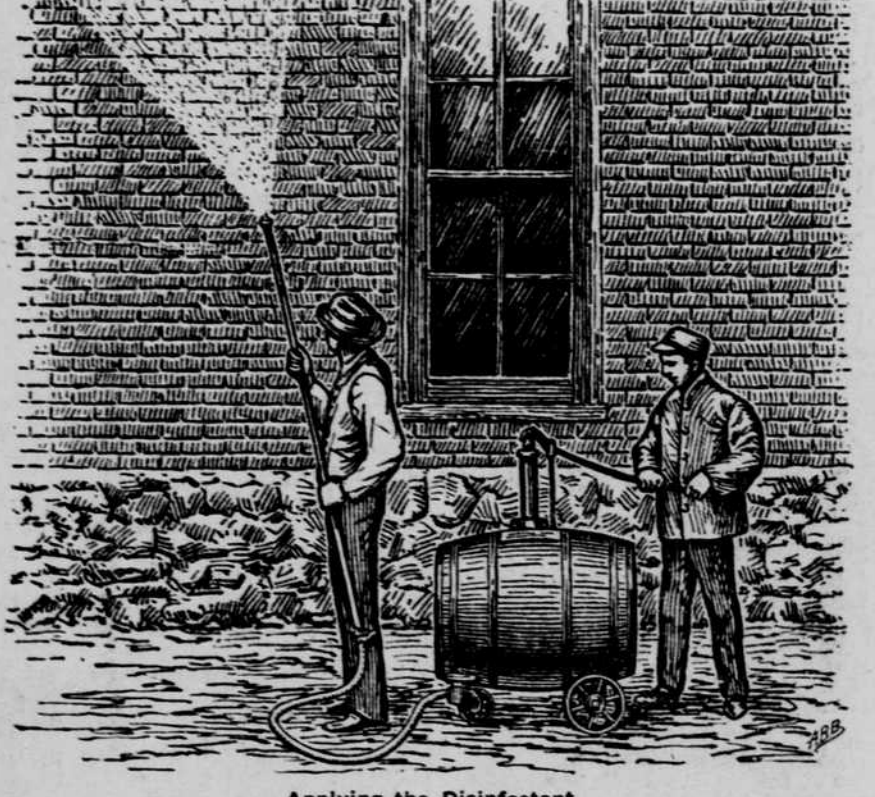
Applying the Disinfectant.
