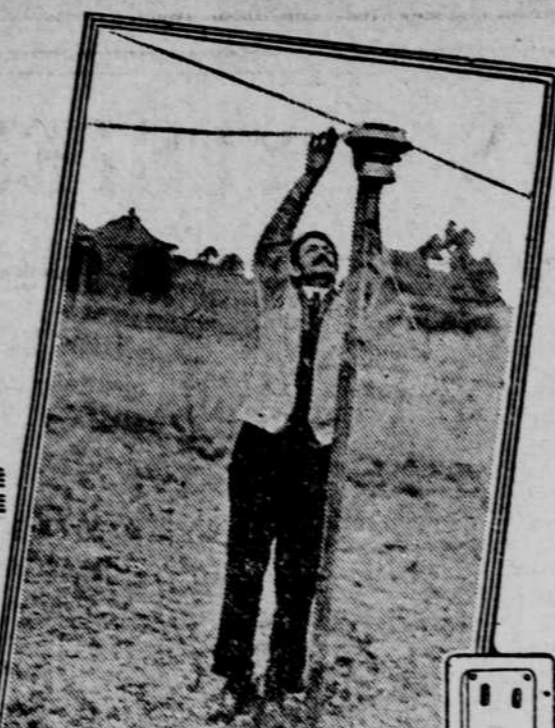
AT WORK ON THE ELECTRIC WIRE ABOVE THE WHEAT AREA
