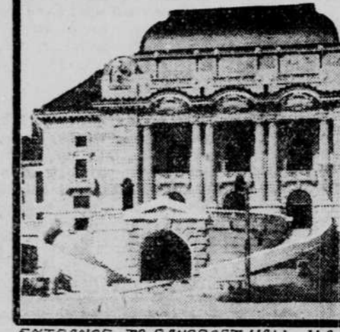
ENTRANCE TO BANCROFT HALL, U.S. NAVAL ACADEMY
