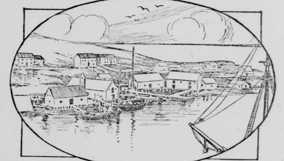
Battle Harbor, Labrador, Showing Two Buildings of the Deep Sea Hospital to the Left.
