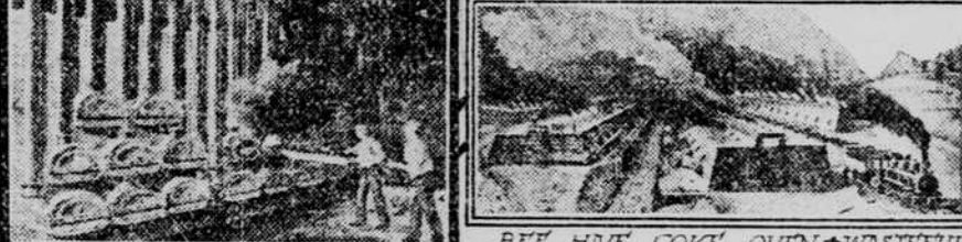
THE NEW COKE OVEN WASTEFUL PROCESS, AS ALL BY-PRODUCTS ARE LOST.
