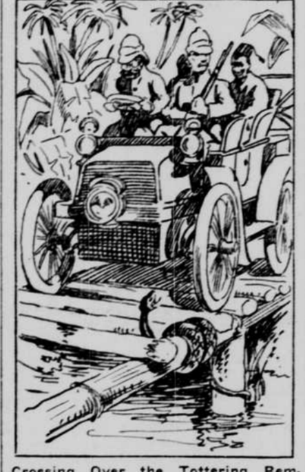
Crossing Over the Tottering Remnants of a Bridge.
