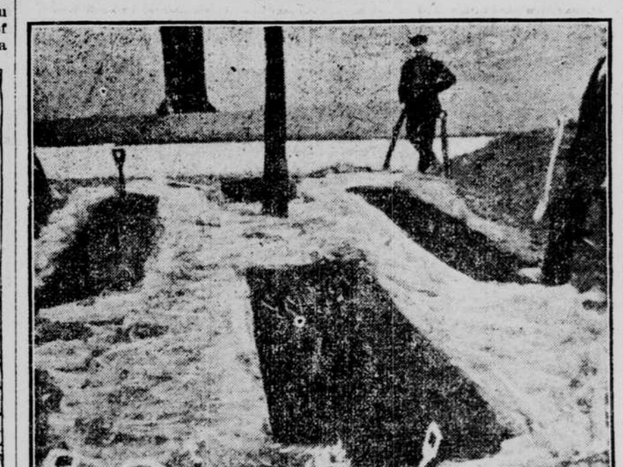
Central Tunnel Made.
