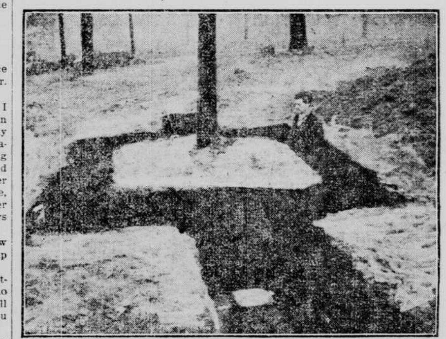
Side Trenches Made.
