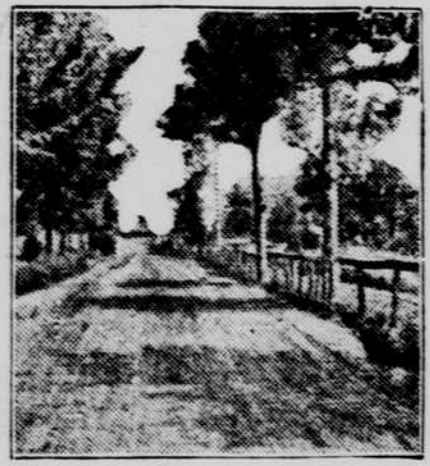
Macadam Road Treated With Asphalt Binder.
