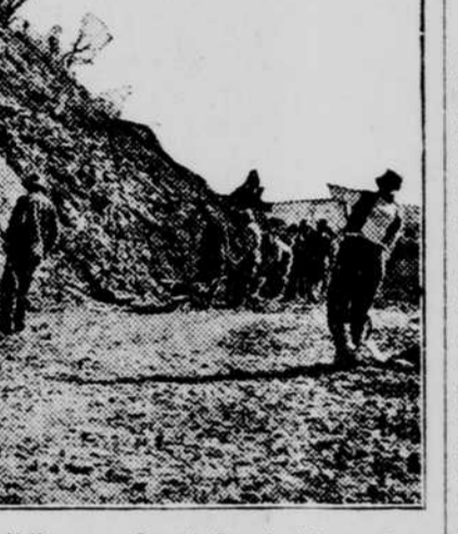
Building a Good Road Through a Hill.
