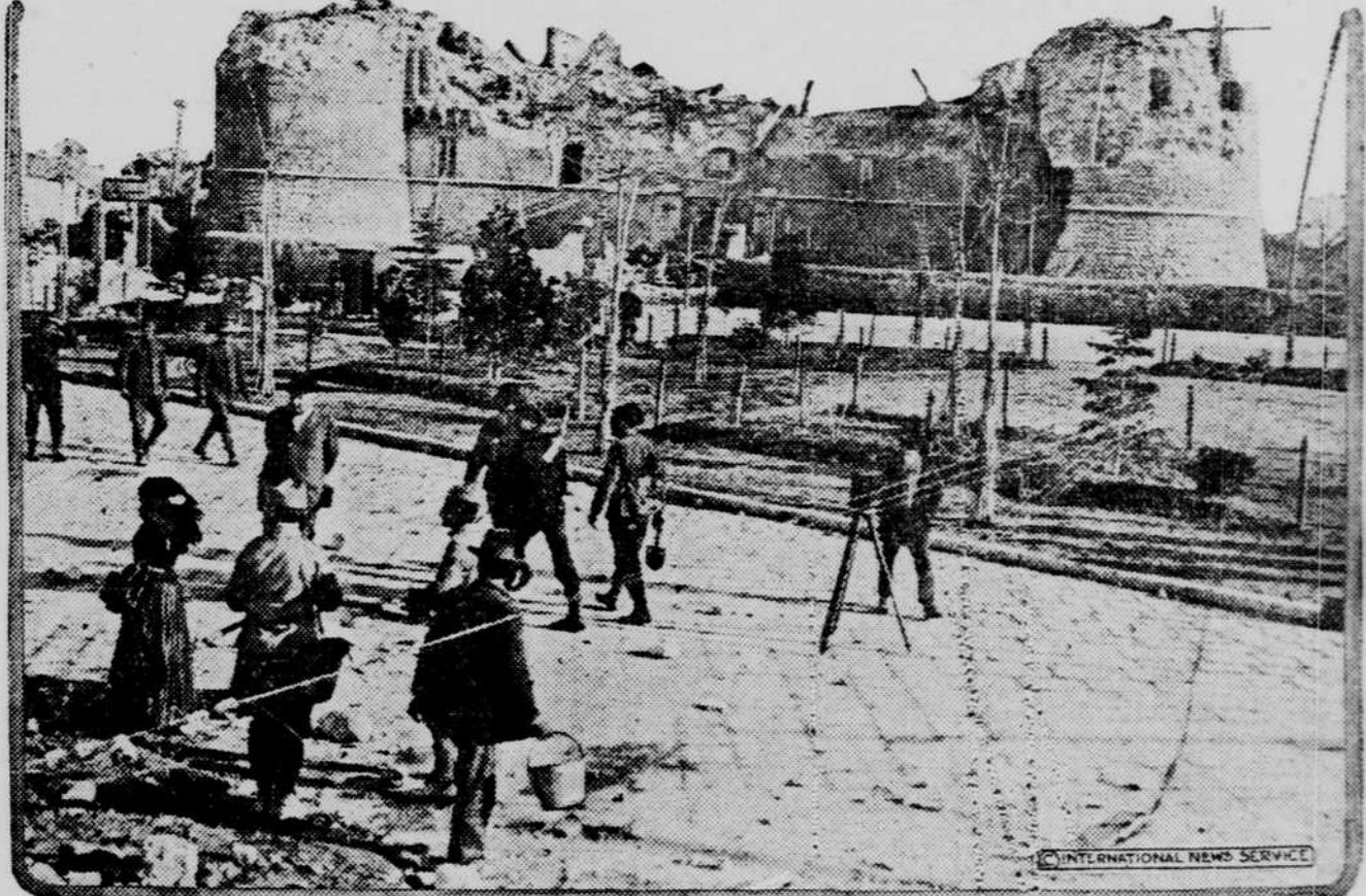
All that was left of the famous Torlonia castle at Avezzano after its massive walls had been shaken down by the recent earthquake in Italy. It was built in 1490.
