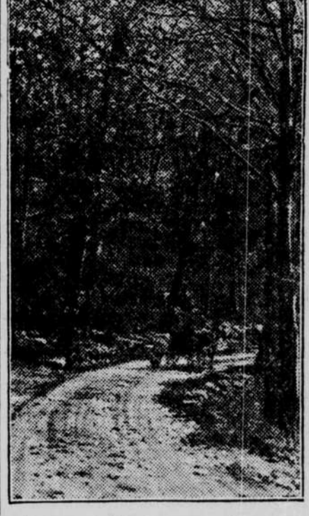
Improved Road in the Woods.
