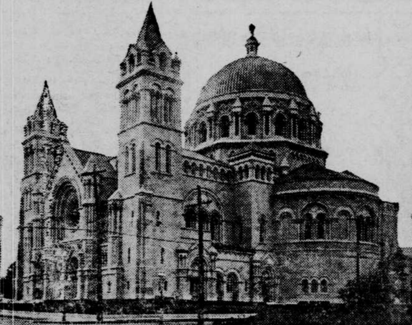
This new Catholic cathedral in St. Louis, just opened, compares favorably in size with the largest church edifices in the world and ranks among the most impressive in America. It is 305 feet long, 212 feet wide, and the main dome is 227 feet high. The seating capacity is 3,500. The cathedral has been under construction six years and so far about $1,500,000 has been spent on it. According to George D. Barnett, the architect, as much more will be devoted to the completion of the interior.
