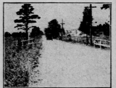
Road Treated With One Application of an Oil Emulsion—Automobile Traveling at Rate of 40 Miles an Hour, With No Dust Resulting.
