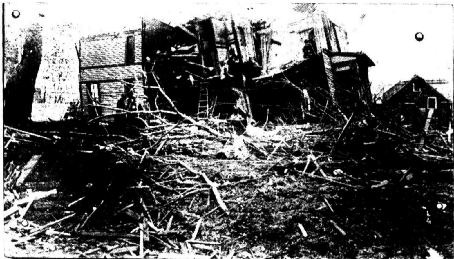
Parmalee Home at Twenty-fourth and Corby, Omaha, as totally demolished by tornado. Those inside escaped under the corner seen at the lower left of the picture. Miss Harriet Parmalee was a well known student of the University last year and a member of Kappa Alpha Theta. Immediately behind the Parmalee wreck in which no one was injured can be seen ruins in which were found four bodies.
