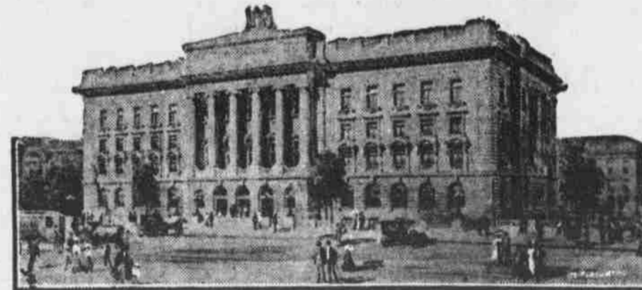
Now under construction, $1,200,000. Court House, Youngstown, Ohio.
