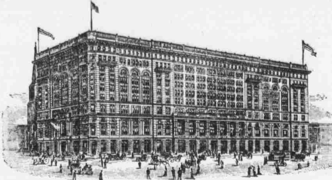
Largest Office Building in the World—Madison Avenue, Fourth Avenue, 23rd Street and 24th Street, New York City.
