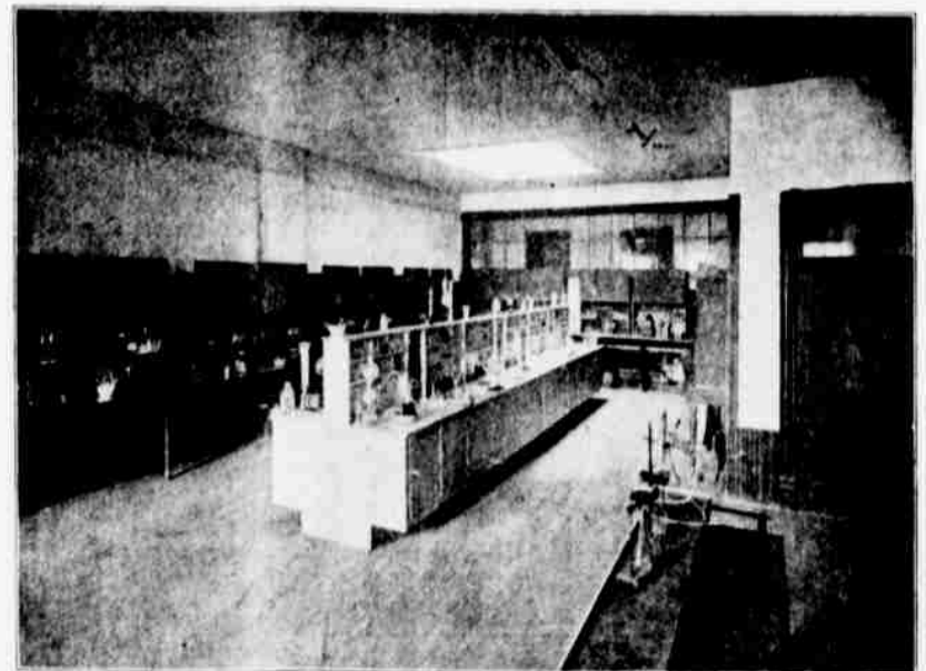
SECTION OF CHEMISTRY ROOM
