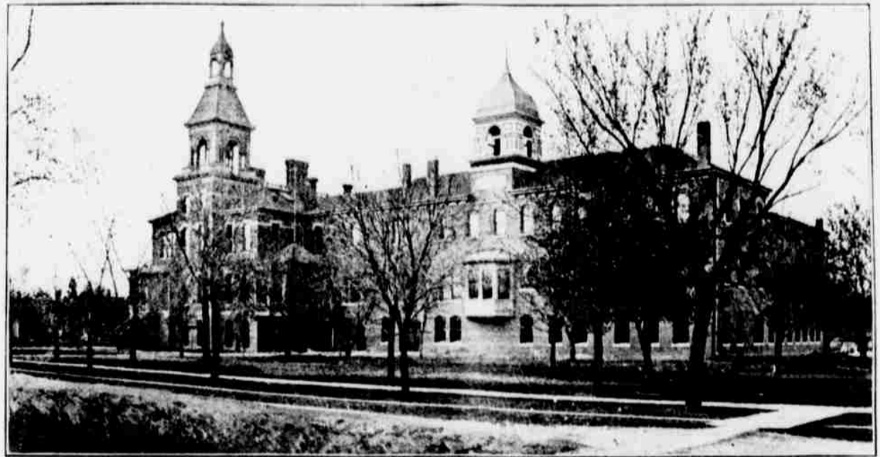
MAIN BUILDING FREMONT NORMAL SCHOOL
