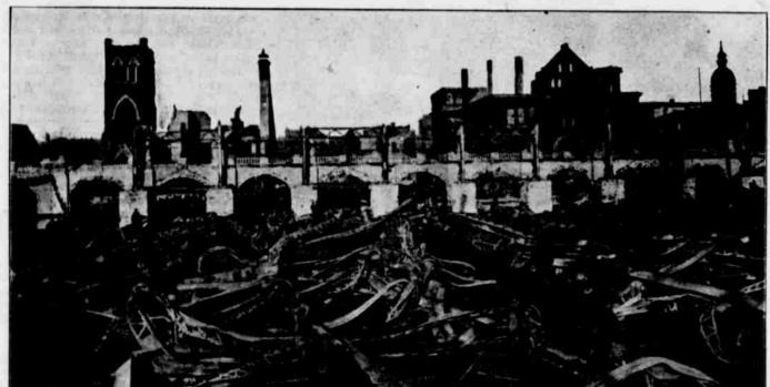
INTERIOR OF BURNED KANSAS CITY AUDITORIUM-SHOWING BENT AND TWISTED STEEL ARCHES.
