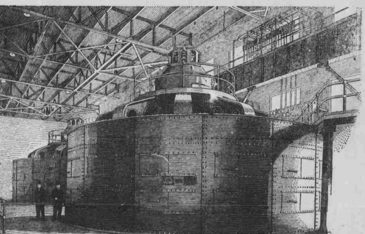
This giant hydro-electric unit weighs 750 tons and consists of a vertical shaft hydraulic turbine attached to an electric generator delivering 52,000 kilowatts at 12,000 volts.
