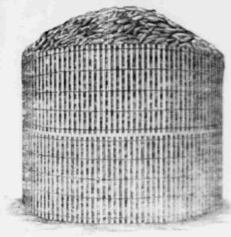
Made with 10 Galvanized Steel Wire Cables around each Crib interwoved with 5c-inch . Pickets, space 1½ inches apart. \* \* \* \* \*
