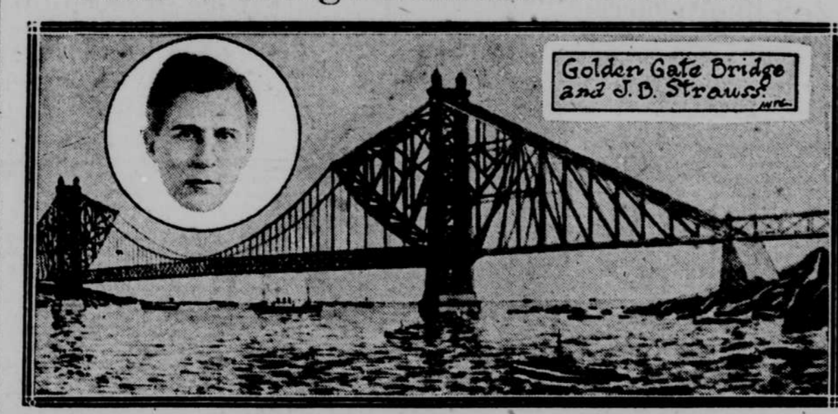
J. B. Strauss, noted Chicago bridge builder, has a plan to bridge the famous Golden Gate in San Francisco with the greatest span in the history of the world. The center would be 4,000 feet long, and the towers higher than Eiffel Tower, in Paris, the tallest structure in the world. The towers would be provided with elevators for sight-seers. The bridge, cantilever and suspension affair, would connect San Francisco and Marin county to the north.
