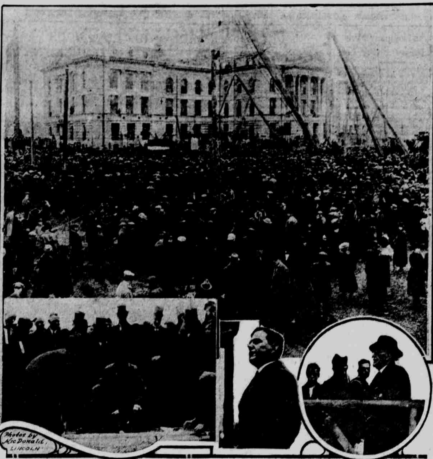
The top picture shows a portion of the crowd of 8,000 Nebraskans who viewed the laying of the cornerstone of the new $5,000,000 state house at Lincoln Armistice day. The picture was taken as the cornerstone was being lowered into position. Below at the left is shown Col. Alvin M. Owsley, national commander of the American Legion, laying the cornerstone of the new capitol, which is dedicated to American fallen soldiers. Below at the center is a picture of Colonel Owsley delivering his dedication address. Below at the right is a picture of Col. J. H. Pruesson of Omaha offering the invocation at the ceremonies.
