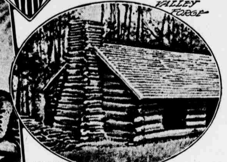
HOSPITAL HUT RESTORED ON VALLEY FORGE CAMP GROUND
