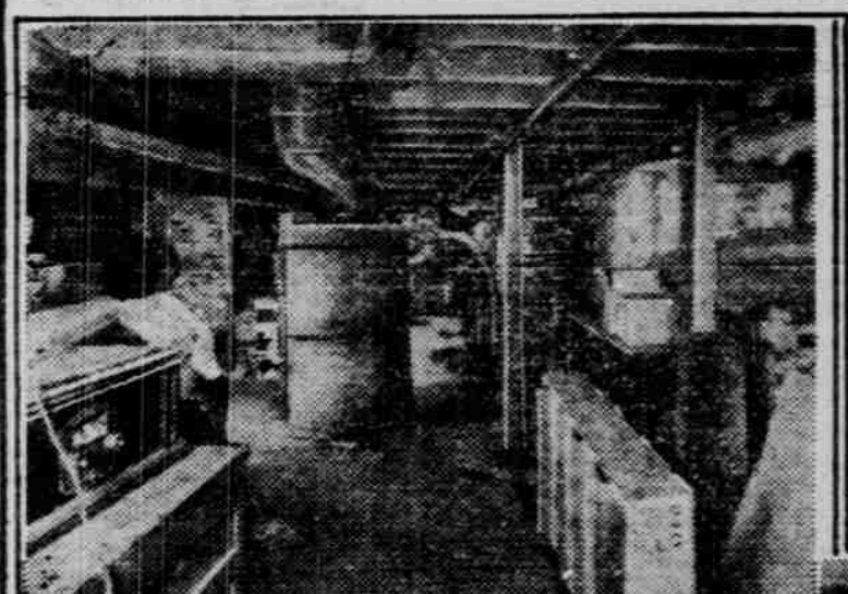
Cellar Reborn— Above you will find what this cellar looked like before it was remade into a children's playroom. Heating is gravity warm water, gas fired. Consumers Information reports a growing tendency to convert unsightly cellars into recreation rooms for adults, home gymnasiums and offices and children's playrooms such as the one shown here.
