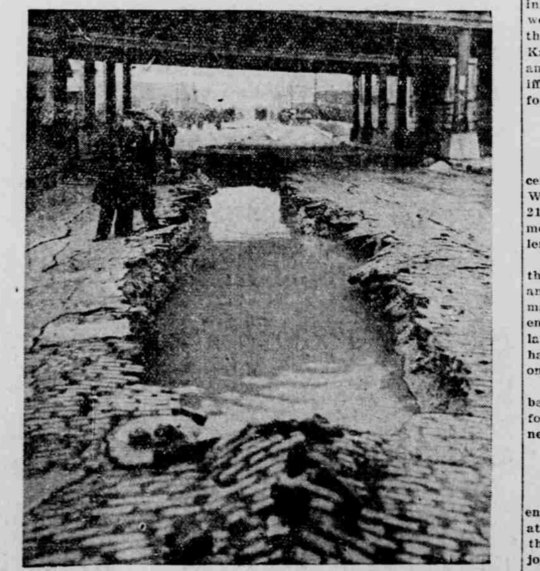
This great water-filled hole in Armitage Avenue, Chicago, was created by one of the terrific subterranean blasts which rocked the Northwest Side of that city Friday, causing serious injury to three persons and property damage estimated at $1,000,000. The explosions are laid to an accumulation of sewer gases.
