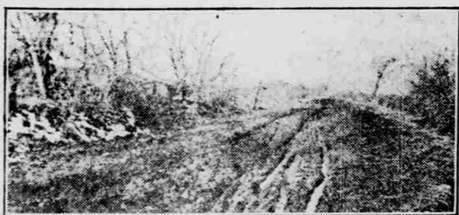
Three-fourths of the state's roads were in this condition two years ago.
