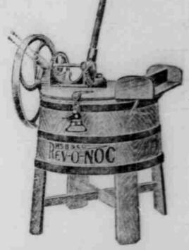
The REV-O-Noc Washing machine is built of cedar, made exceptionally strong and is very easy to operate. The operating lever is so arranged that you may obtain two different positions of handle. Also has fly-wheel in such a position that it may be driven by belt power. For sale only by
