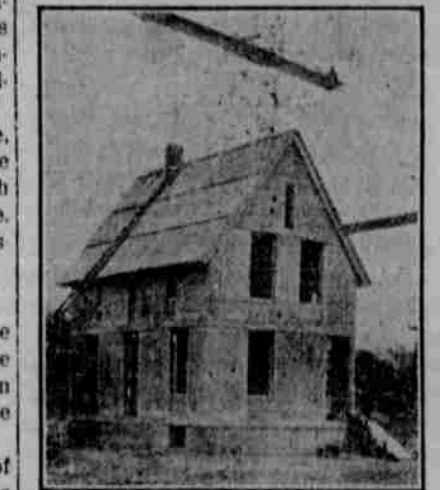
HOUSE MADE OF CEMENT BLOCKS, WITH CRANE USED IN ERECTING IT.
