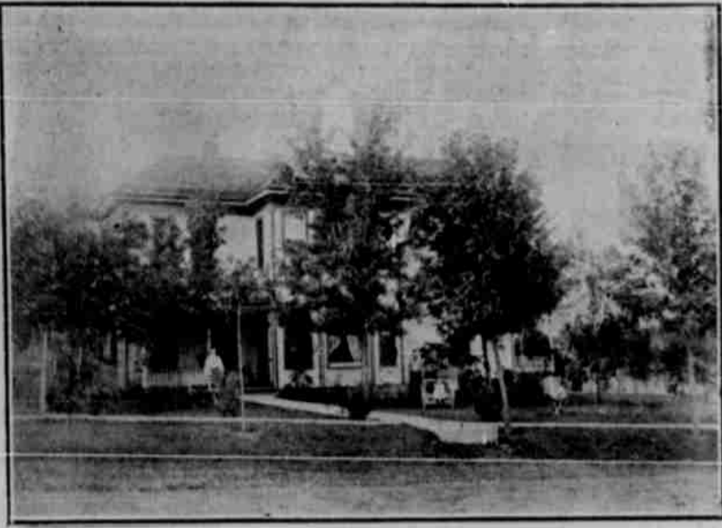
RESIDENCE OF LOUIS W. ROETTGER
