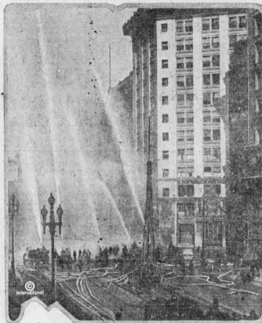
As a last feature of San Francisco's "Safety First" week, the fire department turned on the high pressure system at Third and Market streets, in the heart of the business section. A dozen streams of water shot skyward for hundreds of feet, topping the highest buildings, demonstrating the fact that the city can never again be destroyed by a conflagration similar to the fire of 1906.
