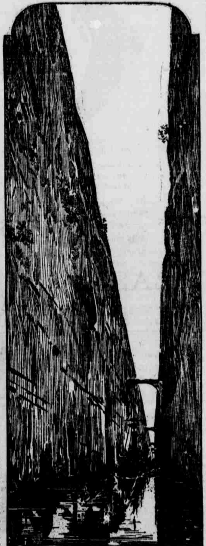
ONE OF THE IMMENSE CUTS THAT WILL BE NECESSARY.
