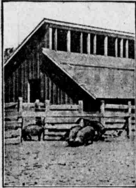
A Well-Constructed Hog House—Provision Has Been Made for Good Ventilation and Sunlight.
