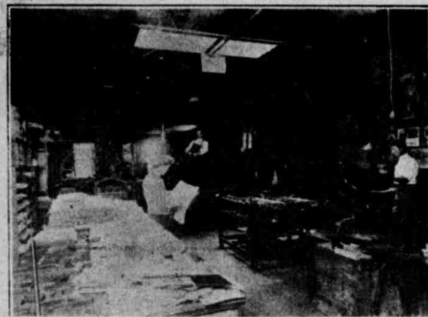
MECHANICAL DEPARTMENT, ALLIANCE HERALD
