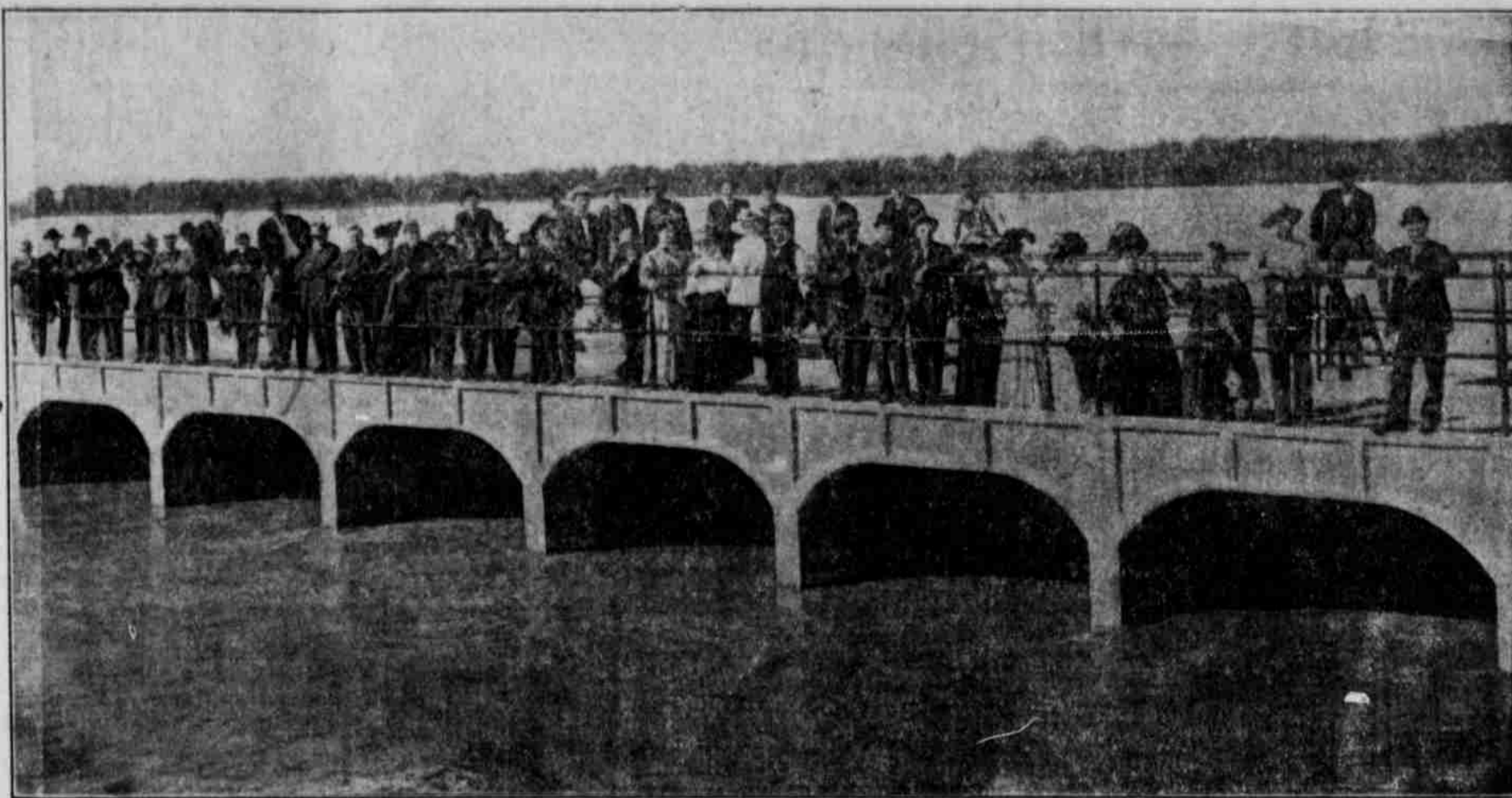
HEADGATES OF ONE OF THE BIG VALLEY CANALS Plenty of Water for Irrigation. The Immense Pathfinder Reservoir in Wyoming Stores One Million Acre Feet
