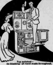
I Standing on the oven door is a very slight test compared with actual use. Malleable frames are absolutely necessary to bear the strain. Any range that will not bear you on its oven door isn't strong enough to stand the test
